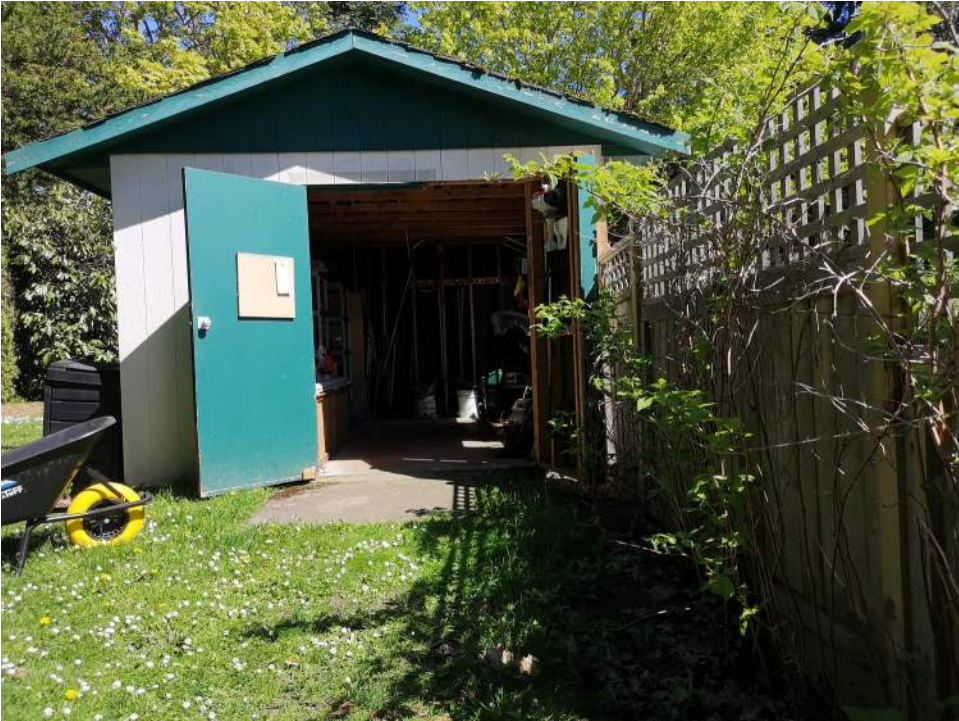
Photo - G20 40 99.01 - Garden Shed / Repair
