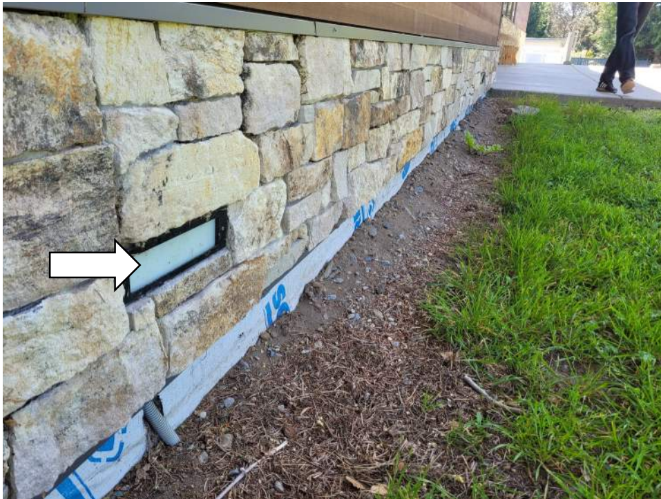
Photo - D40 20 06.01 - Exterior Lighting - Replacement / Rockwall-Mounted at Narthex
