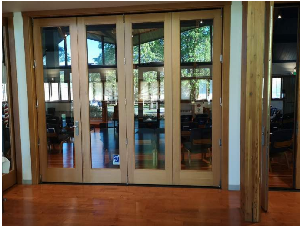
Photo - C10 20 03.02 - Interior Doors - Repairs / Narthex
