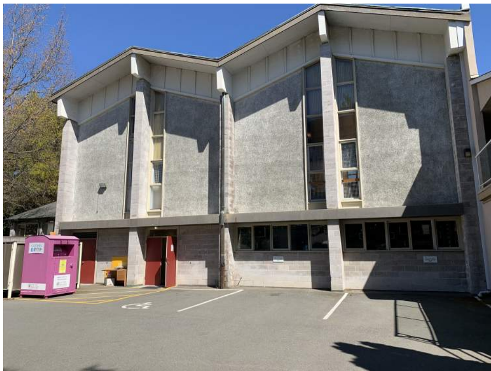
Photo - G20 10 00.01 - Asphalt Pavement - Resurfacing / Parking Areas
