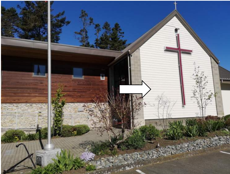
Photo - B20 10 01.03 - Fiber Cement - Exterior Wall - East Elevation / Original Church
