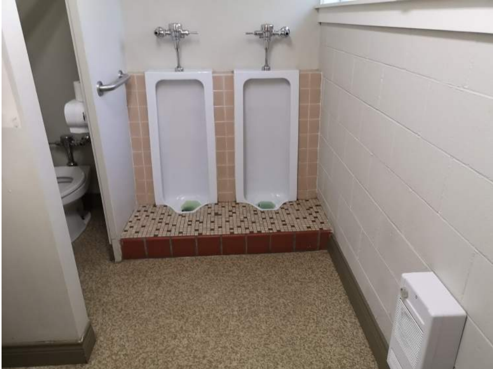
Photo - D20 10 02.01 - Plumbing Fixtures - Replacement / Washrooms
