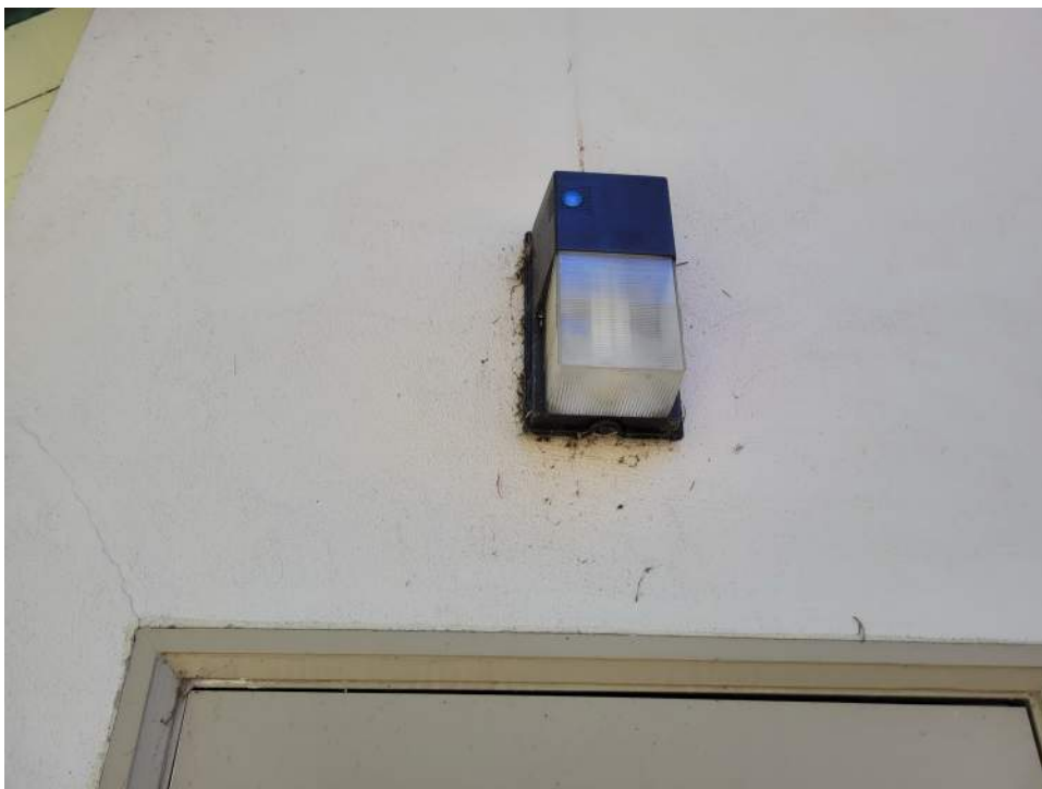
Photo - D40 20 06.02 - Exterior Lighting - Replacement / Wall-Mounted at Church
