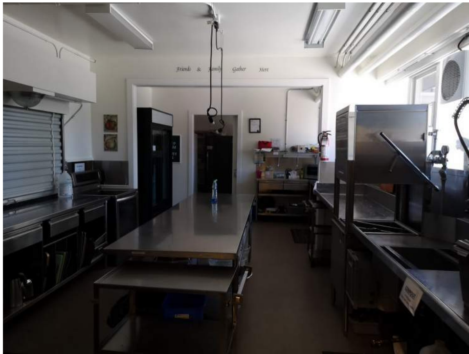
Photo - C30 00 00.04 - Interior Finishes and Furnishings - Refurbishment / Kitchen - Ground Level
