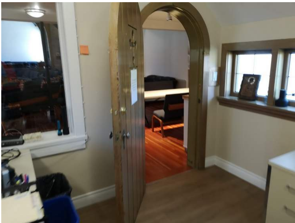
Photo - C10 20 03.01 - Interior Doors - Repairs / Original Church
