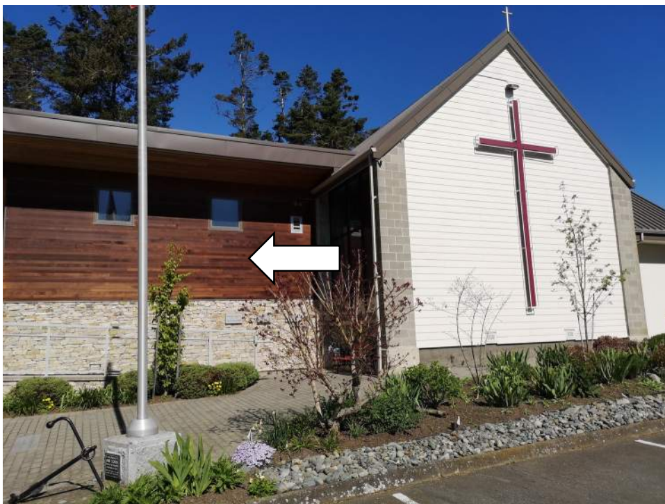
Photo - B20 10 01.05 - Cedar Cladding - Replacement / Narthex
