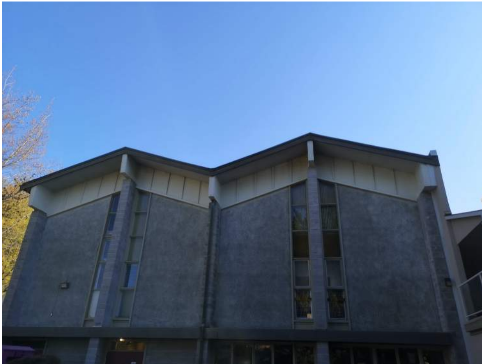
Photo - B20 10 01.01 - Stucco Cladding - Replacement / Exterior Walls
