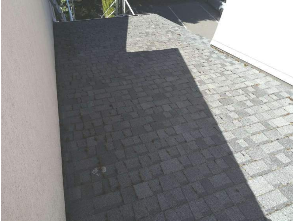
Photo - B30 10 02.02 - Asphalt Shingles - Replacement / Over Southeast Emergency Exit Deck
