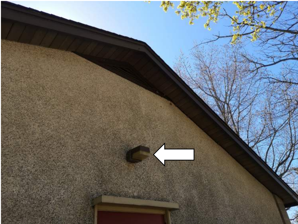
Photo - D50 20 02.02 - Exterior Lighting – Replacement
