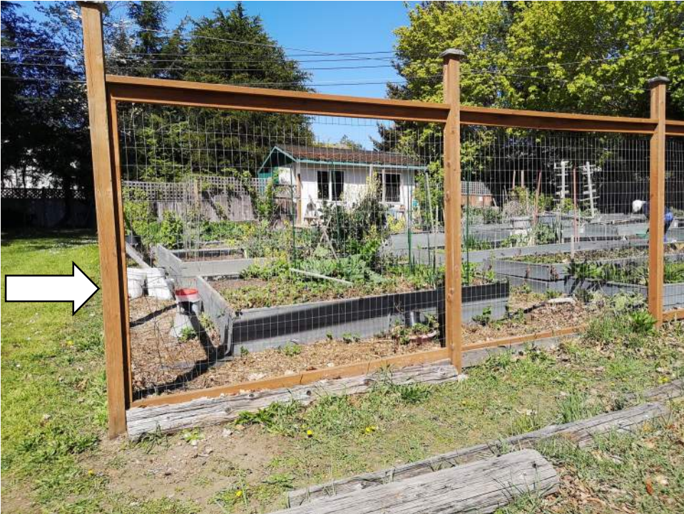
Photo - G20 40 01.02 - Fences - Replacement / Around Garden Beds
