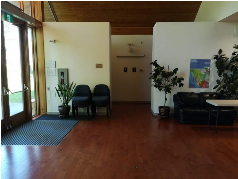
Photo - D40 30 03.00 - Fire Alarm System - Replacement / Throughout
