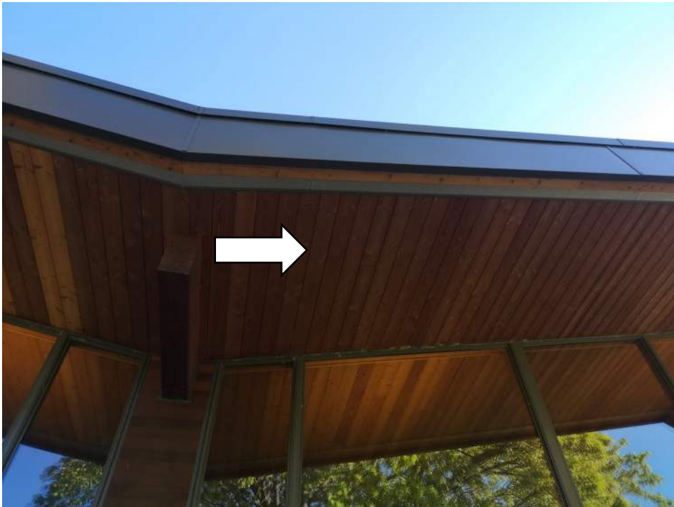
Photo - B20 10 08.02 - Soffits - Restain and Repair / Roof Overhangs / Narthex
