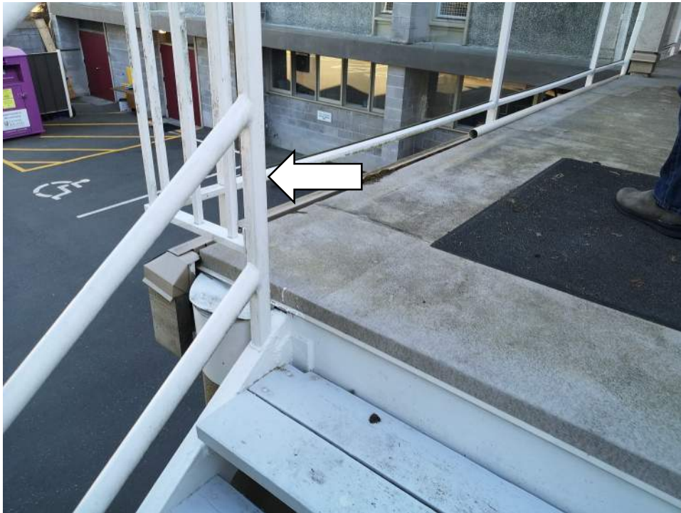
Photo - B10 10 04.02 - Balcony, Guardrails - Replacement/ Southeast Corner of Building
