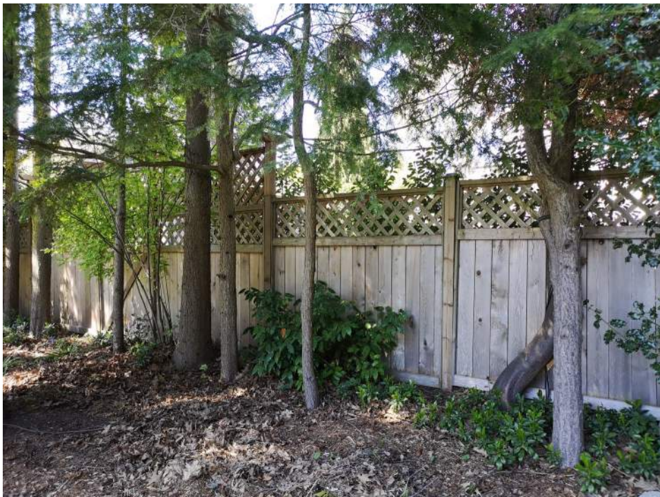
Photo - G20 40 01.01 - Fences - Replacement / Site Perimeter
