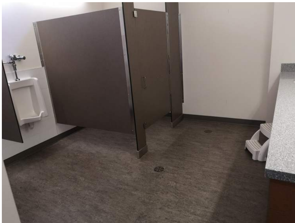
Photo - D20 10 00.00 - Plumbing Fixtures - Replacement / Common Area Washrooms
