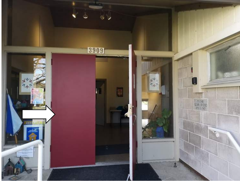
Photo - B20 30 02.00 - Metal Swing Doors - Entrances / Replacement
