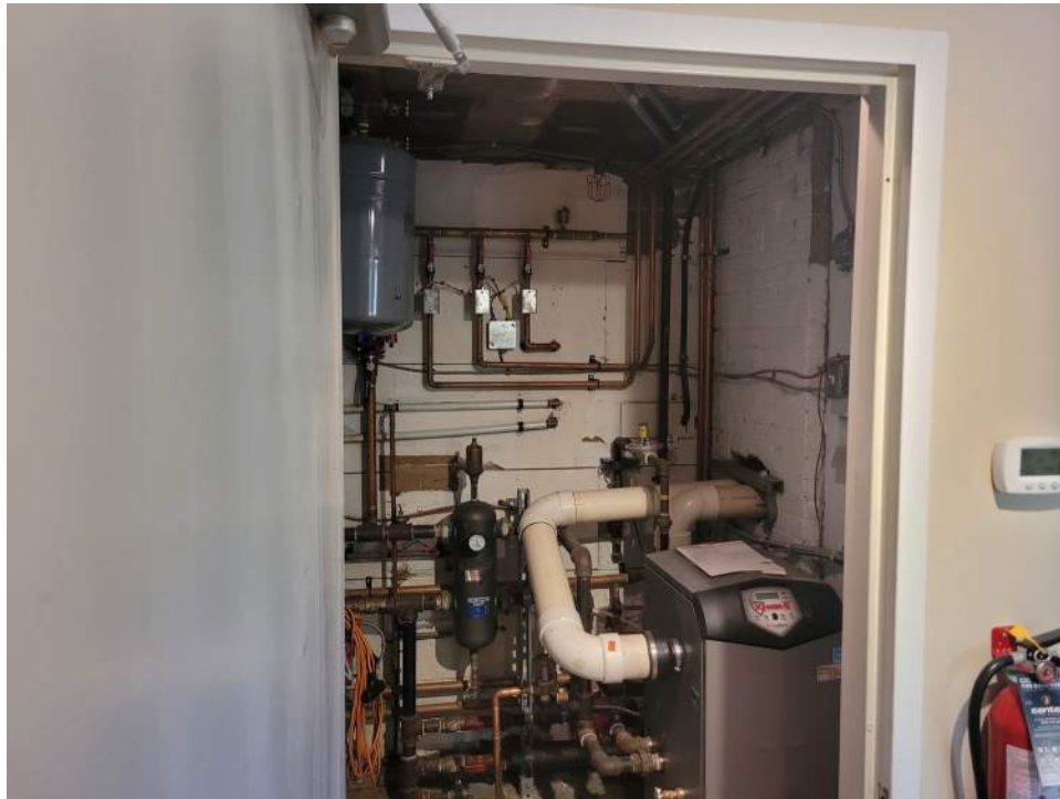
Photo - D20 20 30.00 - Boiler - Replacement / Church Boiler Room
