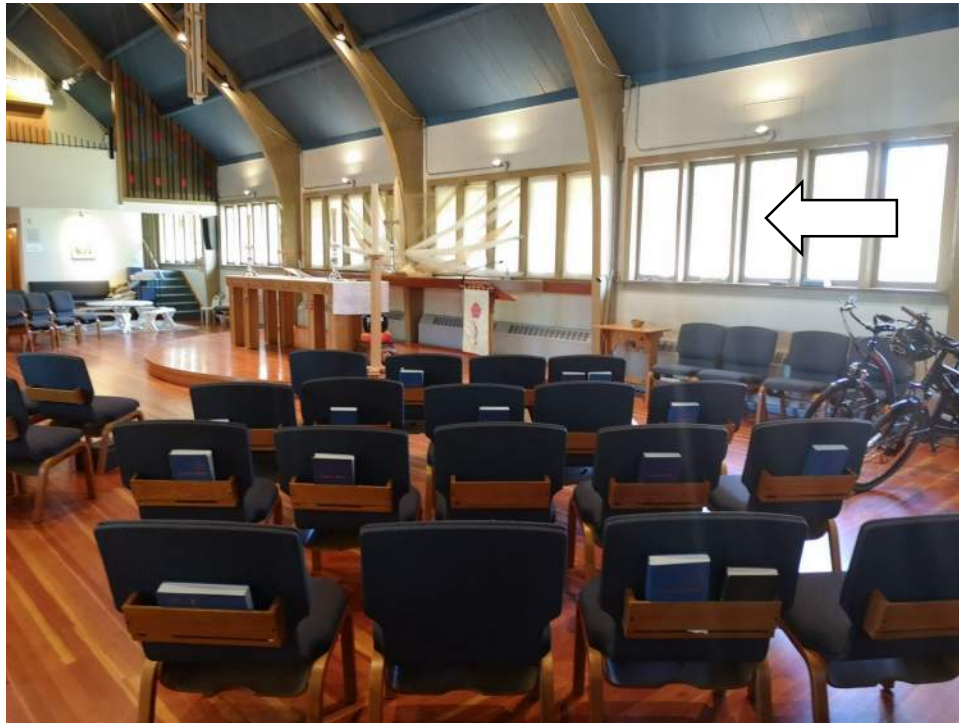
Photo - B20 20 01.03 - Exterior Windows, Wood-Framed - Replacement / Original Church
