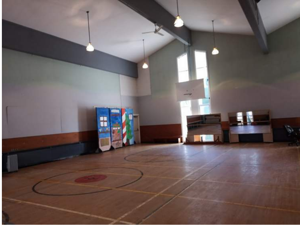
Photo - C30 00 00.03 - Interior Finishes and Furnishings - Refurbishment / Gymnasium
