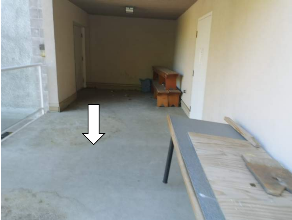
Photo - B10 10 04.01 - Balcony, Vinyl Waterproofing - Replacement / Southeast Corner of Building
