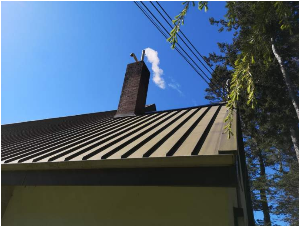
Photo - B30 10 01.01 - Standing Seam Metal Roof - Replacement / High Slope Roof Coverings
