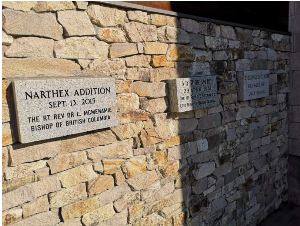
Photo - B20 10 01.07 - Stone Cladding - Replacement / Narthex
