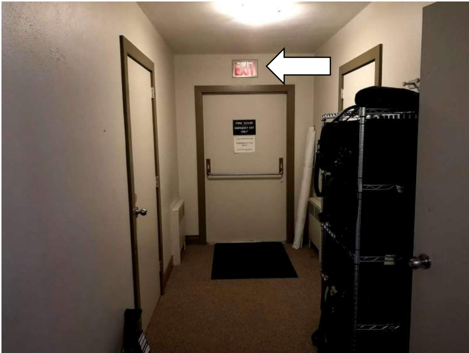
Photo - D50 20 99.00 - Emergency Lighting - Replacement
