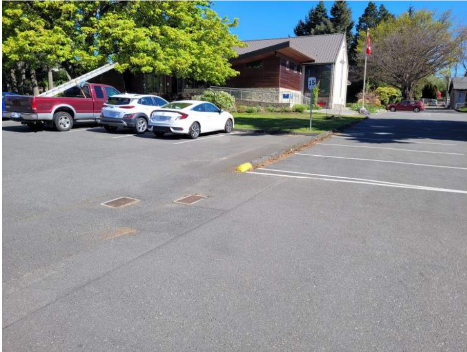
Photo - G20 20 03.01 - Asphalt Pavement - Resurfacing / Parking Areas
