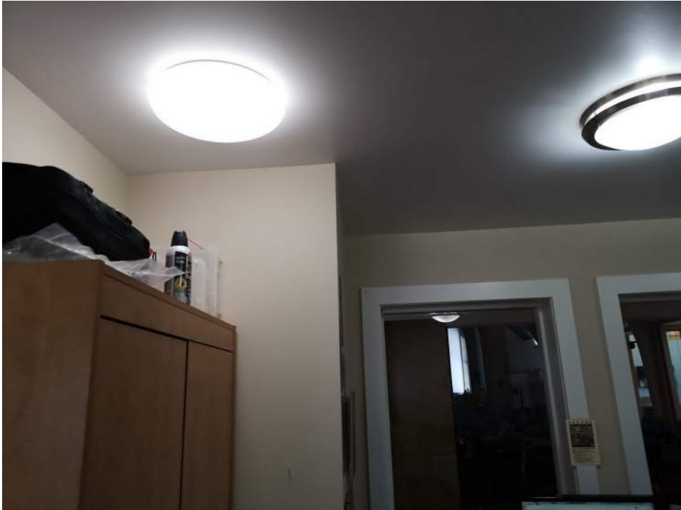
Photo - D40 20 02.01 - Interior Lighting - Replacement / Original Church
