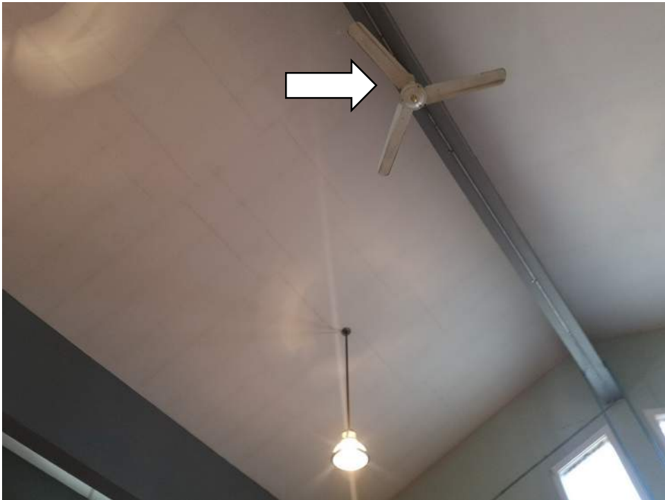
Photo - D30 30 02.00 - Ceiling Fans - Replacement / Gymnasium
