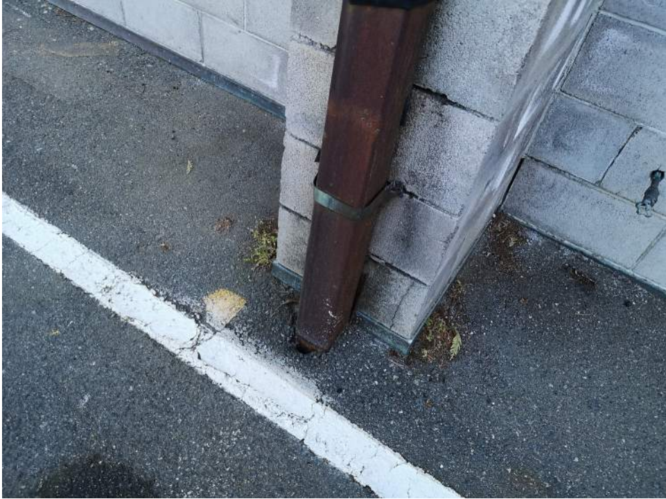
Photo - D20 30 00.03 - Storm Water - Eavestroughs and Downspouts / Around Building
