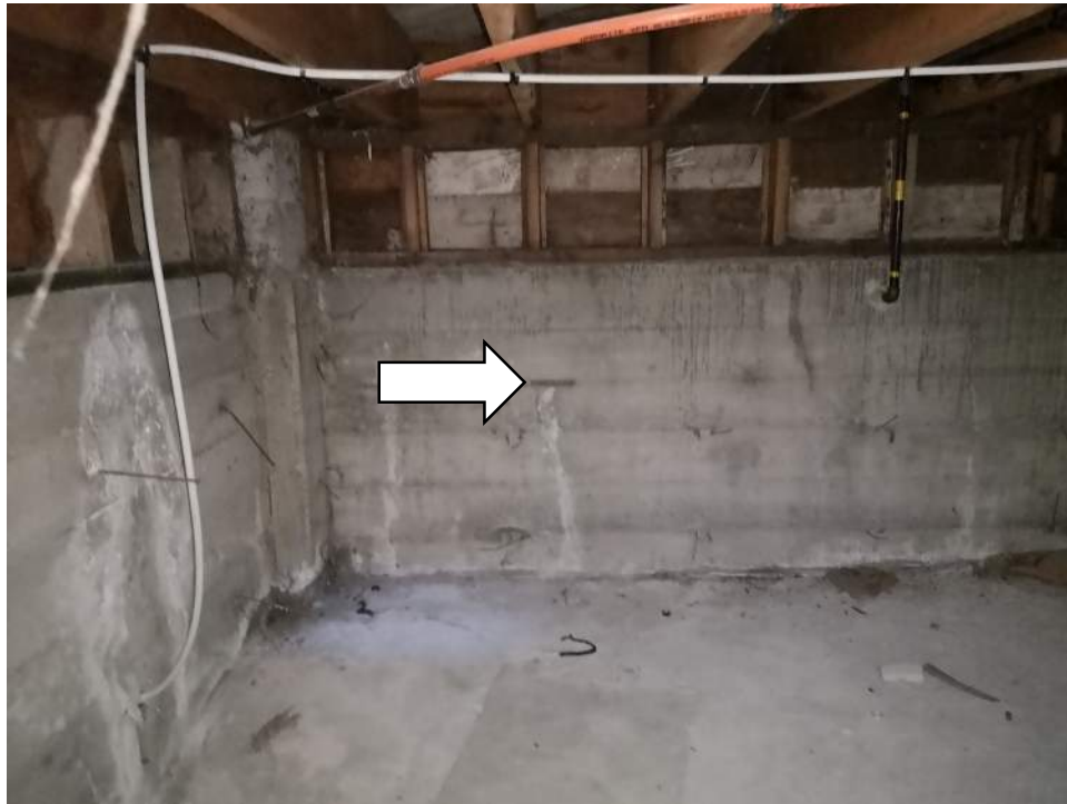
Photo - A10 00 00.01 - Foundations / Below-Grade
