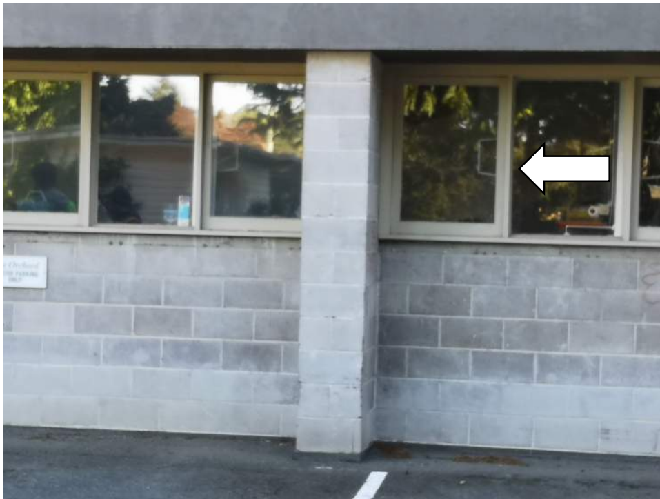
Photo - B20 20 01.01 - Exterior Windows, Wood-Framed - Replacement / Throughout Building Elevations
