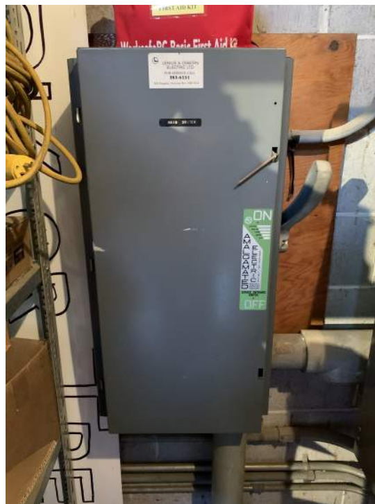
Photo - D50 10 03.01 - Main Distribution Equipment - Replacement / Hall Boiler Room - Kitchen
