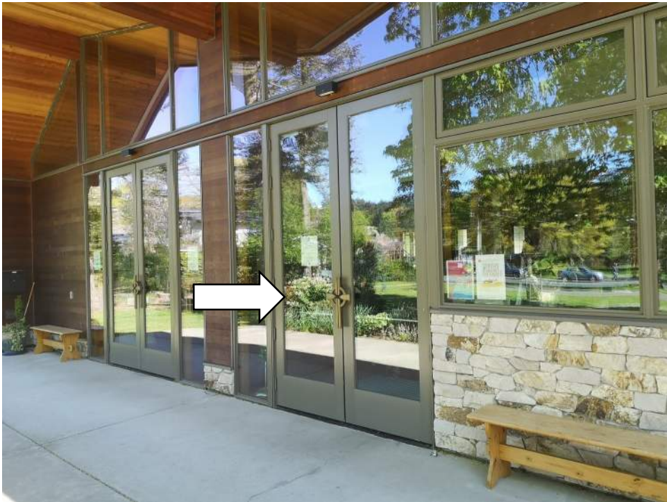
Photo - B20 30 02.00 - Glazed Swing Doors - Replacement / Narthex Entrance
