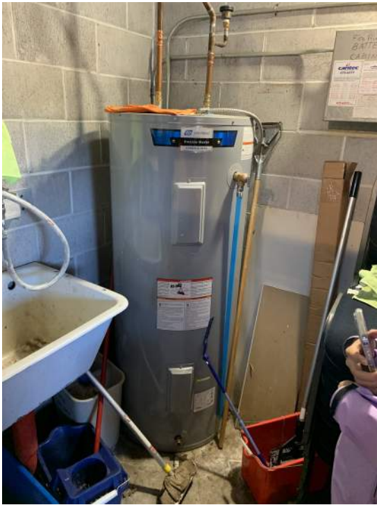
Photo - D20 20 31.00 - Water Heater Tank - Replacement / Hall Boiler Room
