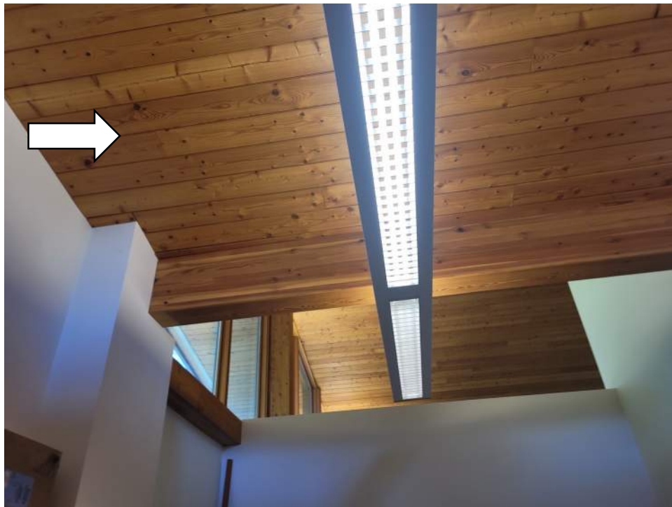
Photo - C30 00 00.08 - Interior Finishes and Furnishings - Stained Shiplap Board Ceiling / Narthex
