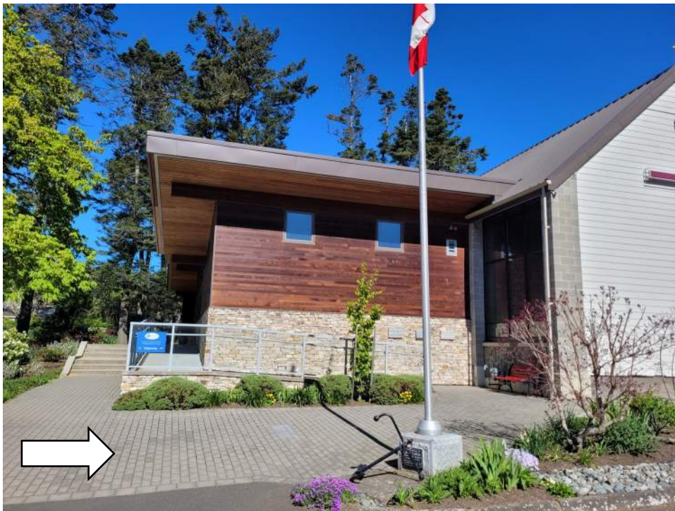
Photo - G20 30 03.01 - Hard Landscaping - Concrete / Walkways and Patios / Front of the Building
