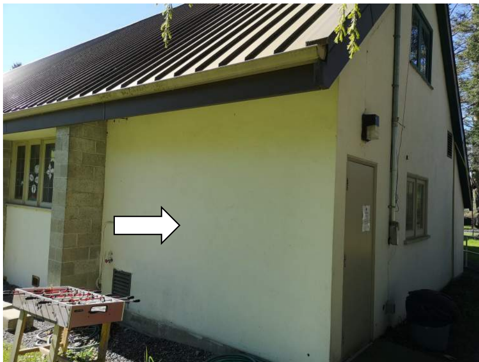
Photo - B20 10 01.01 - Stucco Cladding - Exterior Walls / Original Church
